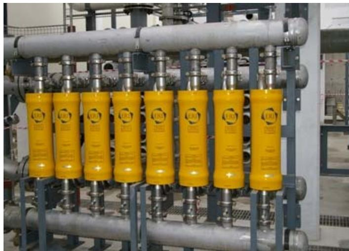
Figure 7 – ERD array with frame for 8 PX units in parallel
