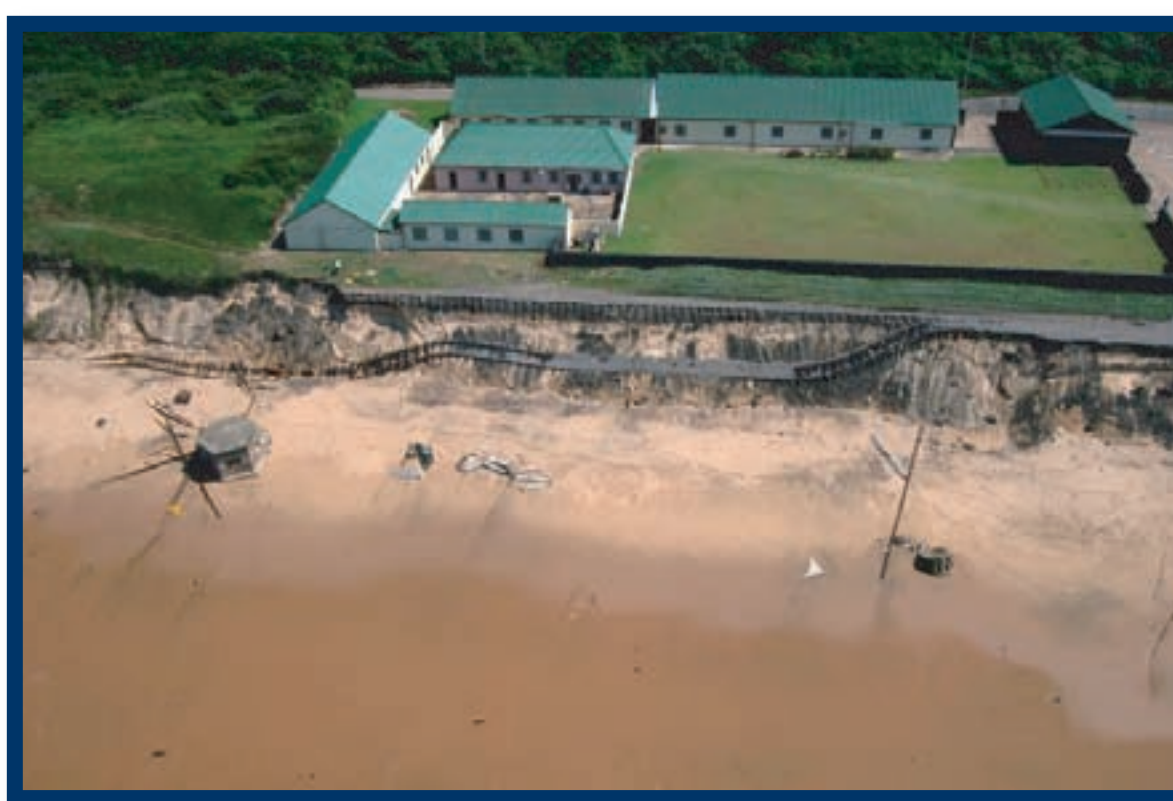
Figure 3: Present SA example of railway line located too close to sea. (Photo: D Phelp)
